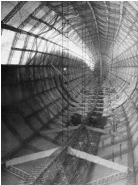
Fig. 8 Inside the hull of the L30, looking forward, after application of the outer cover, but before the gas cells were in place 30) .
